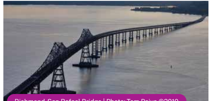
Richmond-San Rafael Bridge | Photo: Tom Paiva ©2010
